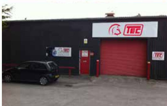
TEC Wales Warehouse
