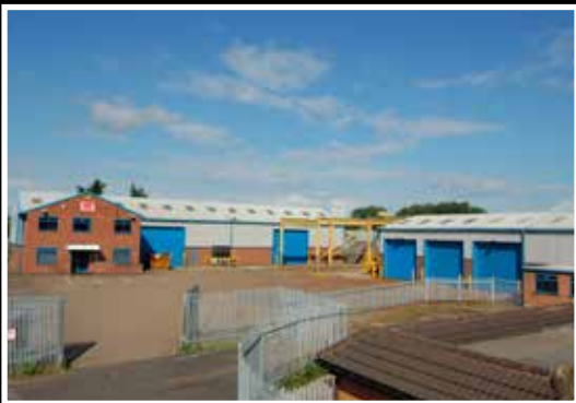
Additional offices and specials division
